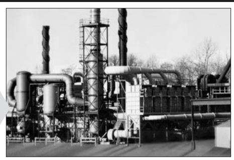
T he lead is processed and smelted in the reverberatory furnace, producing metal which goes to the refinery. There it is placed in kettles, combined with reagents, and alloyed into lead for use in new batteries.
