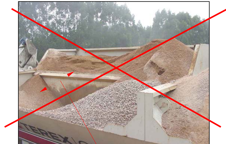
Silo com material contaminado. Silo with contaminated aggregate
