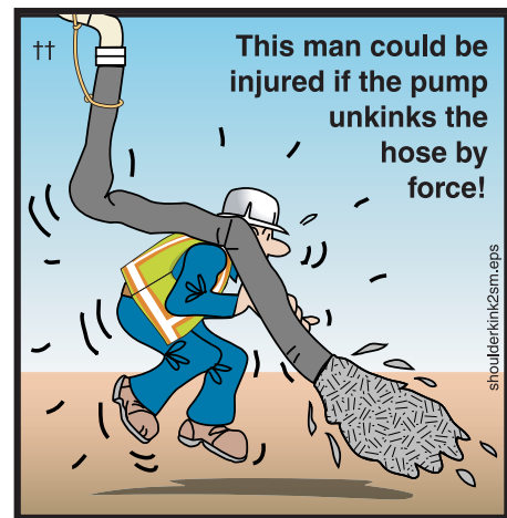
Figure 54 Kinking the hose creates a hazard
