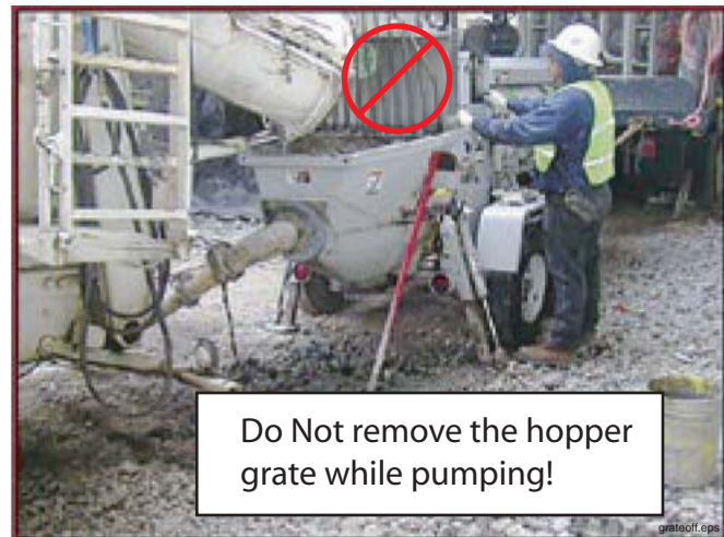
Figure 24 Never remove the hopper grate while the pump is operating
