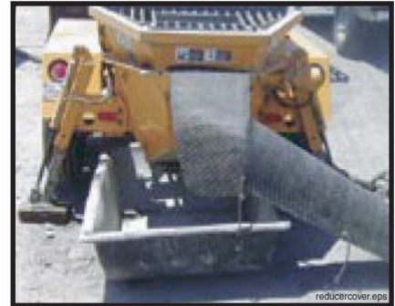
Figure 23 Cover reducers and use containment boxes for cleanout
