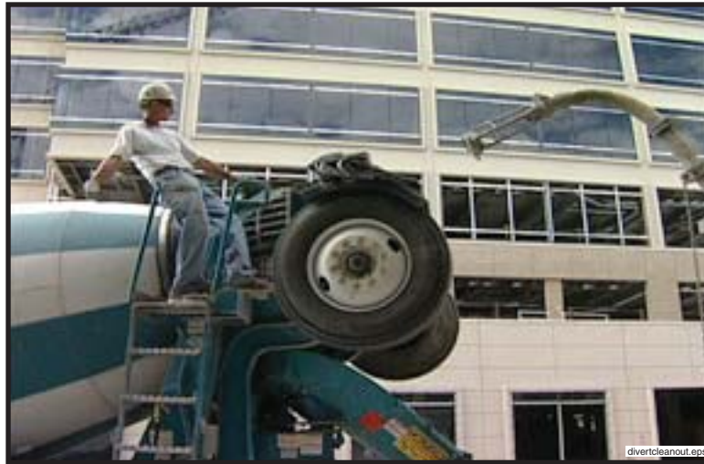
Figure 32 Divert vertical pipeline to the cleanout area and be sure to secure the discharge before continuing
