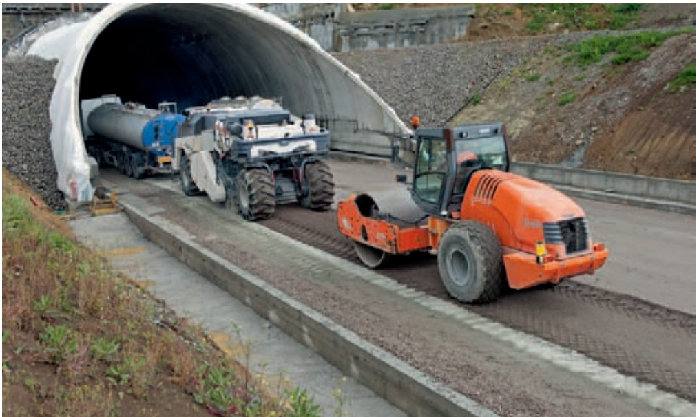
Modern Wirtgen cold recycler WR 240i being used for recycling
